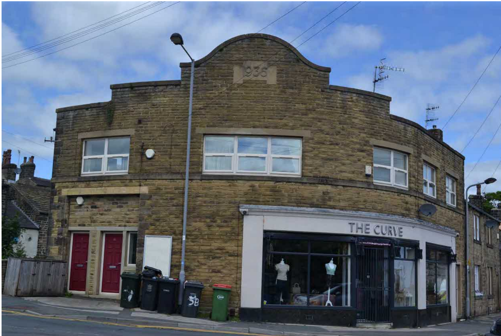
Figure 9. The Curve, built from natural stone.
