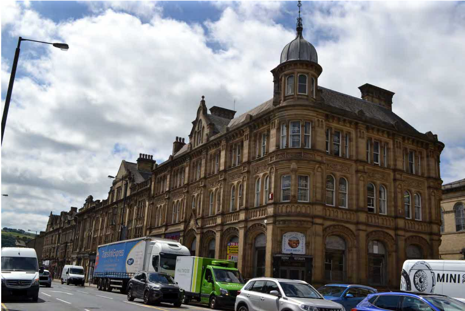
Figure 7: The west side of North Street is constructed from natural stone
