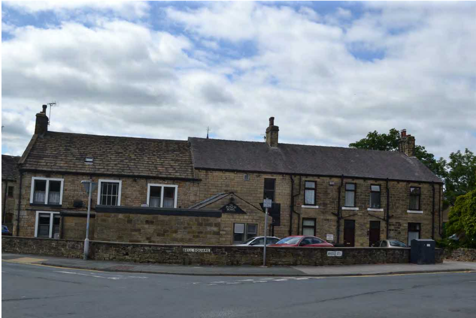
Figure 12. The Punch Bowl viewed from the north, built from natural stone.
