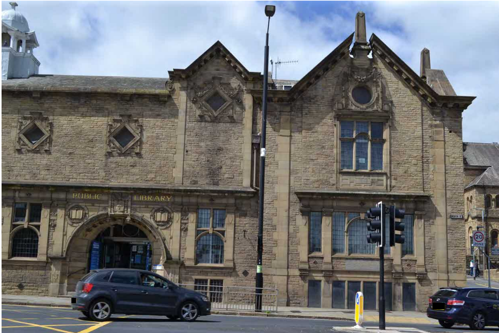
Figure 10: Keighley Public Library is built from natural stone
