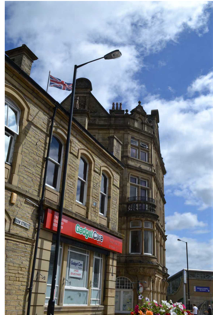
Figure 3: Northern side of Bow Street, buildings constructed from natural stone.
