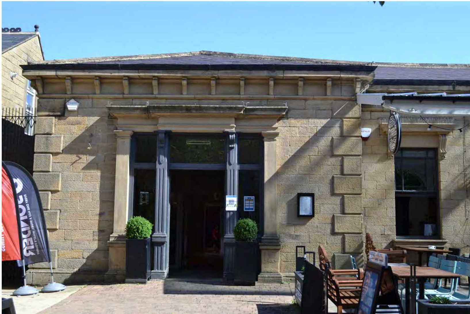
Figure 18: Ilkley Station viewed from the south, constructed from natural stone.
