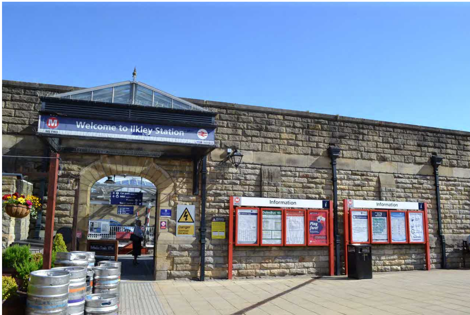
Figure 19: Ilkley Station viewed from the south, constructed from natural stone.
