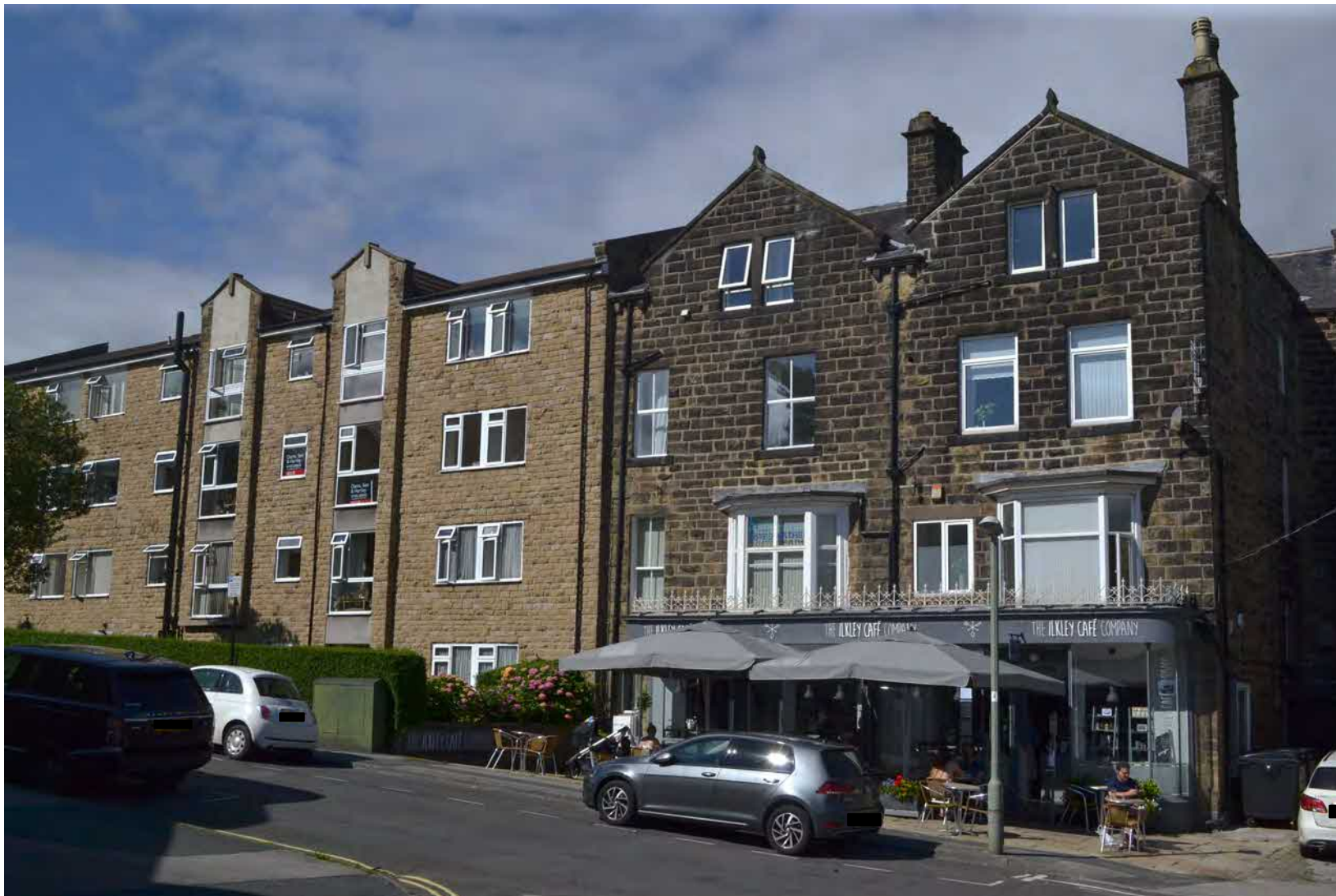
Figure 21: Wells Road viewed from the east. The terrace on the left of the picture is a newer development and has utilized reconstituted stone. The terrace on the right of the picture is older and has been constructed using natural stone.
