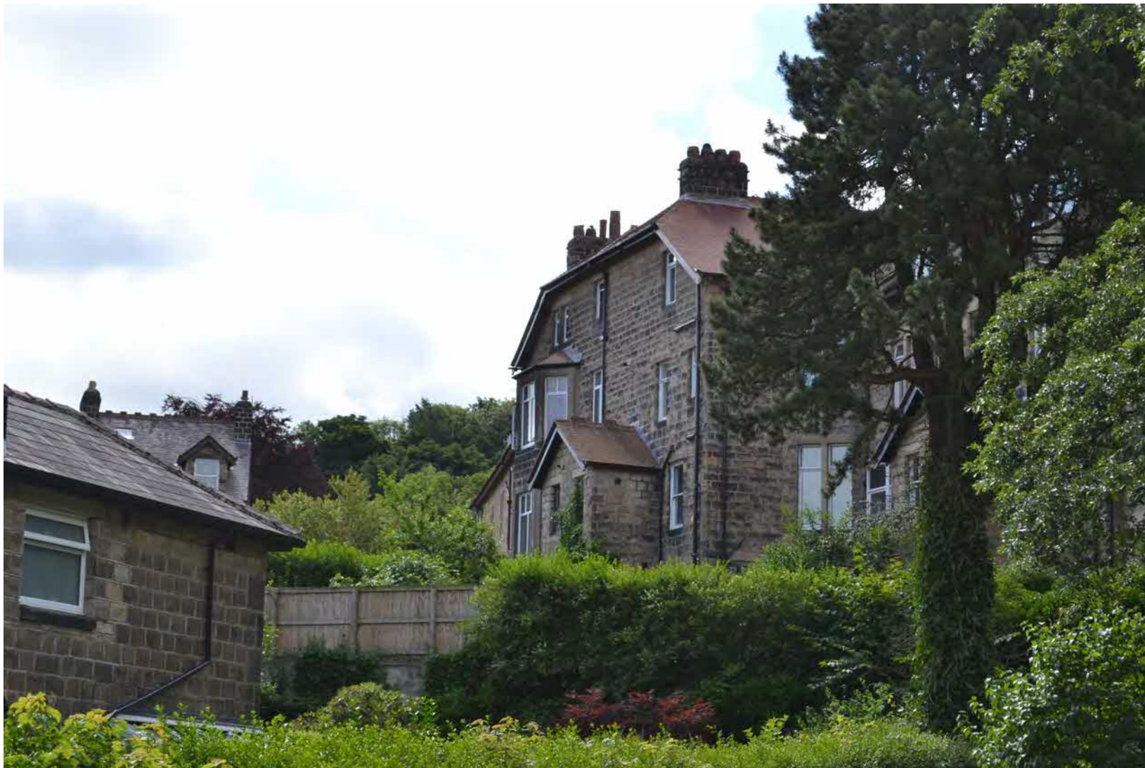
Figure 6: Wilton Road viewed from the south. Houses built from natural stone.
