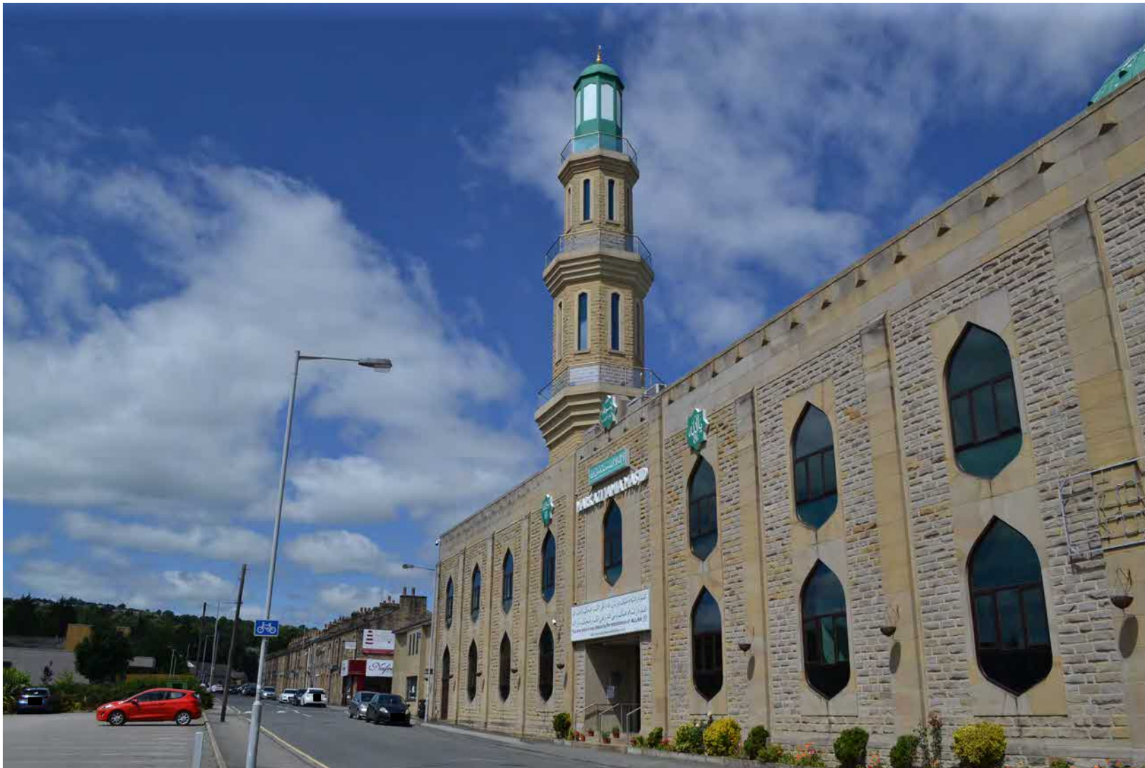
Figure 15: The Markazi Jamia Mosque has been built using natural stone
