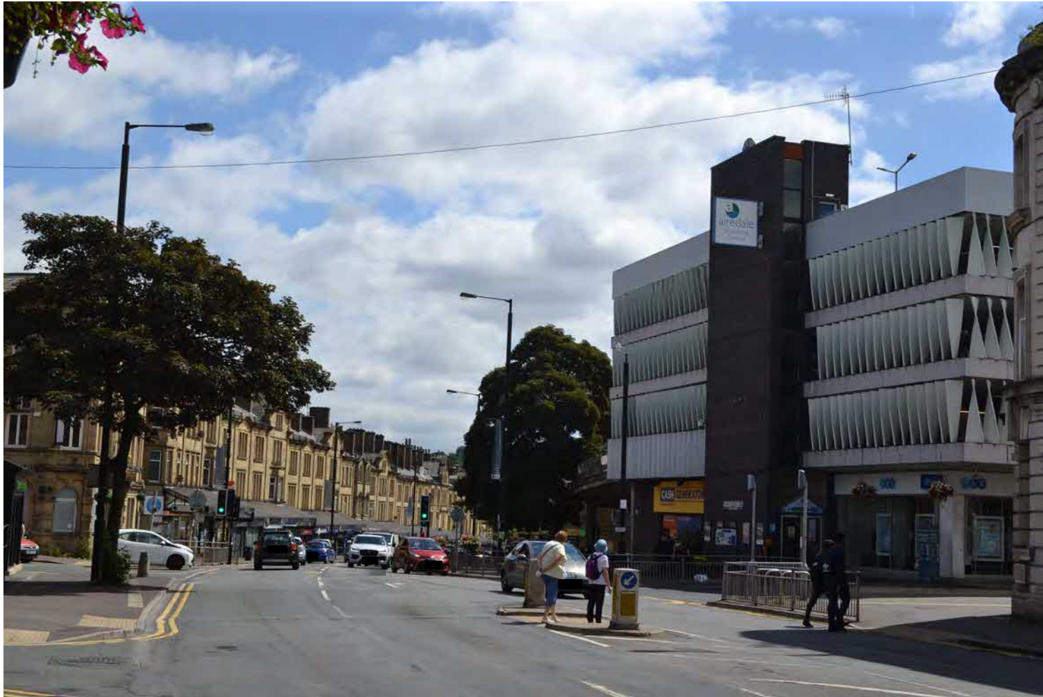
Figure 1: Cavendish Street viewed from the west. The northern side of the street, on the left, is constructed from natural stone. southern side of the street has utilized alternative building materials.
