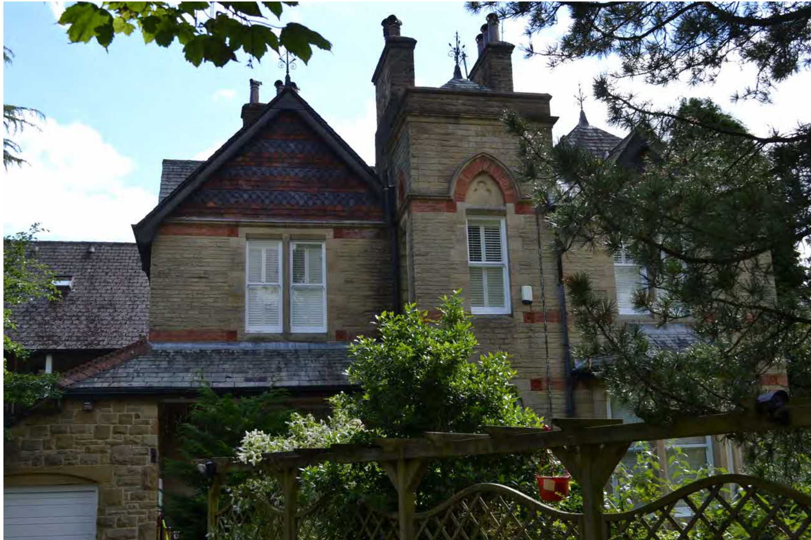
Figure 3: S. Western side of Parade East 3. House built from natural stone with brick and tile details.
