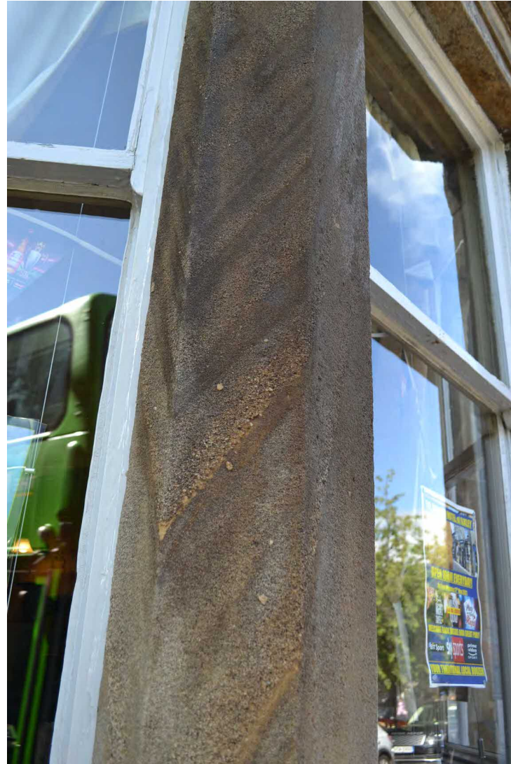
Figure 17: Close-up of the gritstone detail of the Midland Hotel
