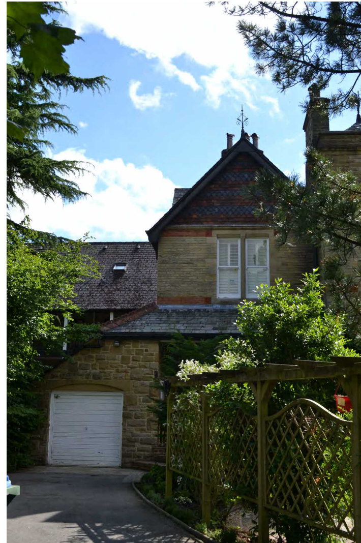
Figure 5: Western side of Parade East 3. House built from natural stone with brick and tile details.
