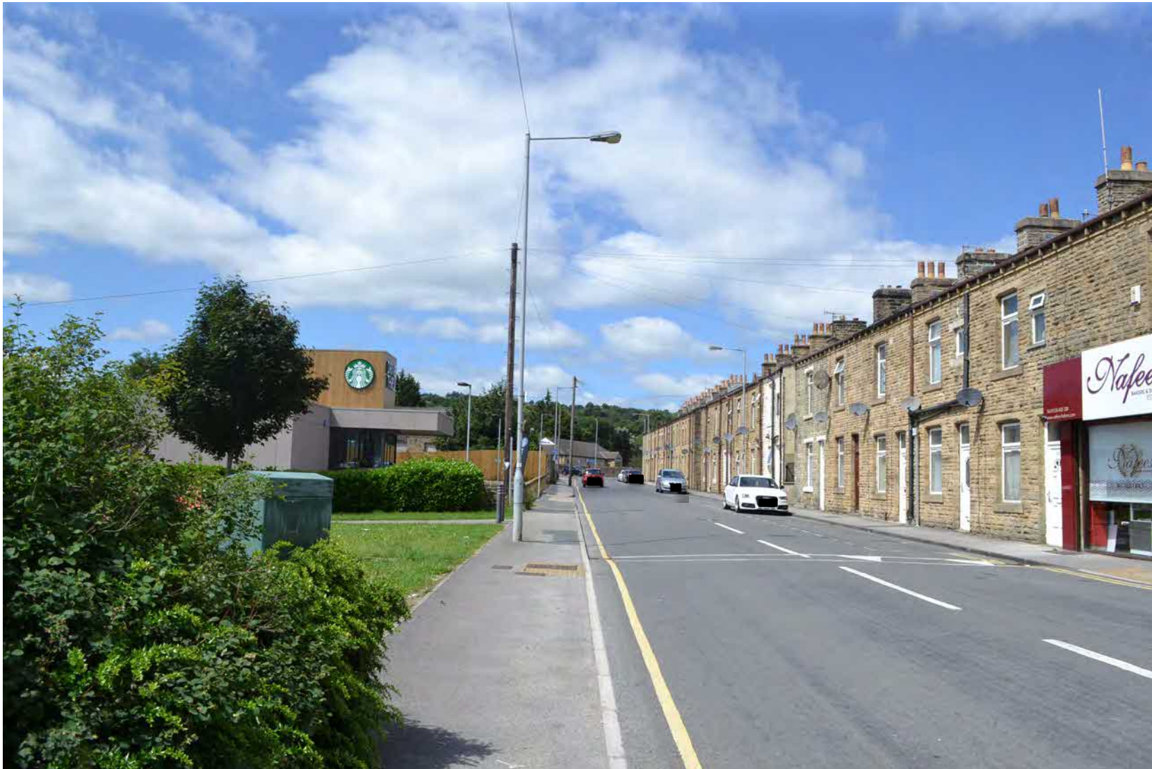
Figure 14: Bradford Street viewed from the west, terraces on the north of the street are built from natural stone.
